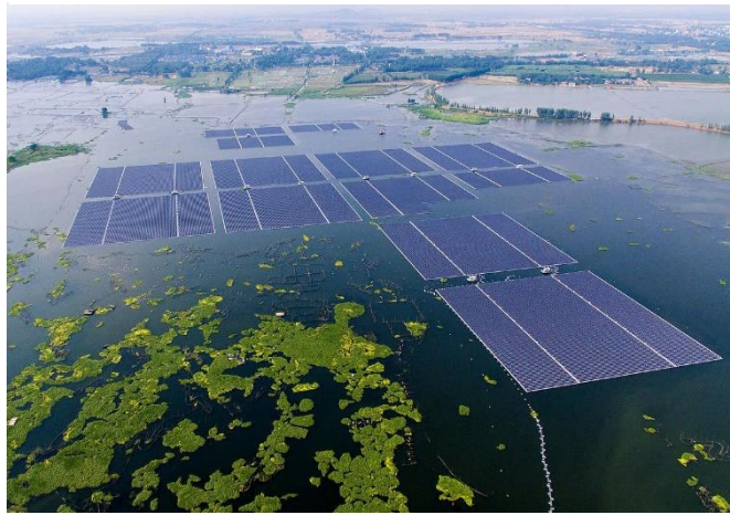
Figure 8: Floating Solar Panels on the Mekong
