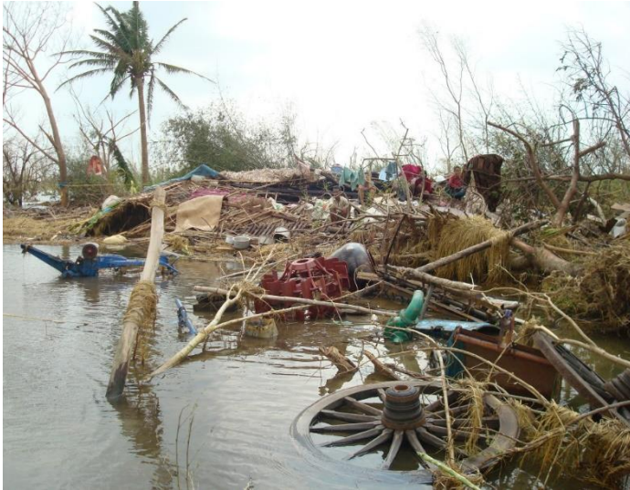
Figure 13: Damage caused by Cyclone Nargis in 2008
